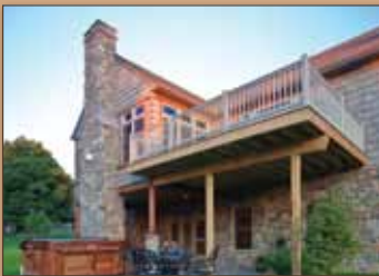
New Construction, Residential, Interior & Exterior – “One & Two Family Dwelling” Merv Miller Spec House Quality Stone Veneer
