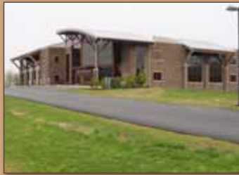
New Construction, Non-residential, Exterior – “Office” J.D. Eckman Corporate Office Eldorado Stone
