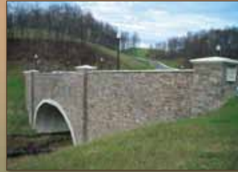
Infrastructure Hardscape/ Landscape WV Bridge Quality Stone Veneer
